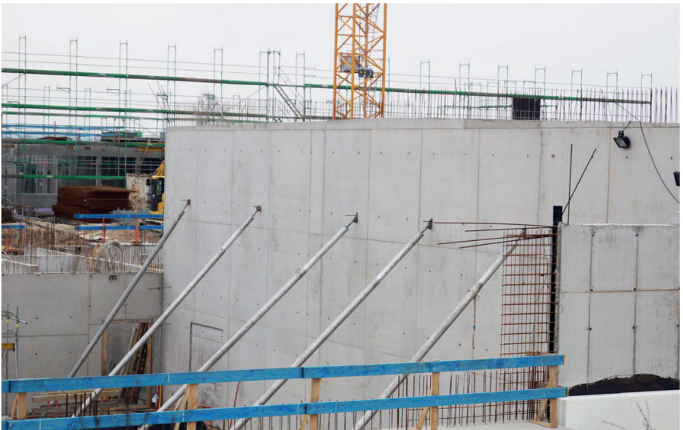
Fastening of guardrails, scaffolding or formwork props
